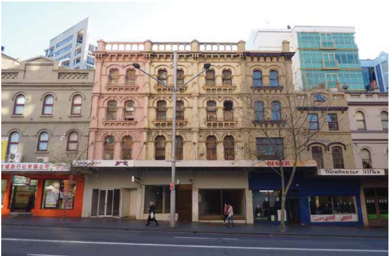
Figure 59 Heritage building - George Street South
